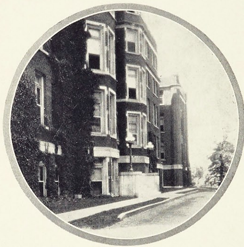
A View of Administration Building
