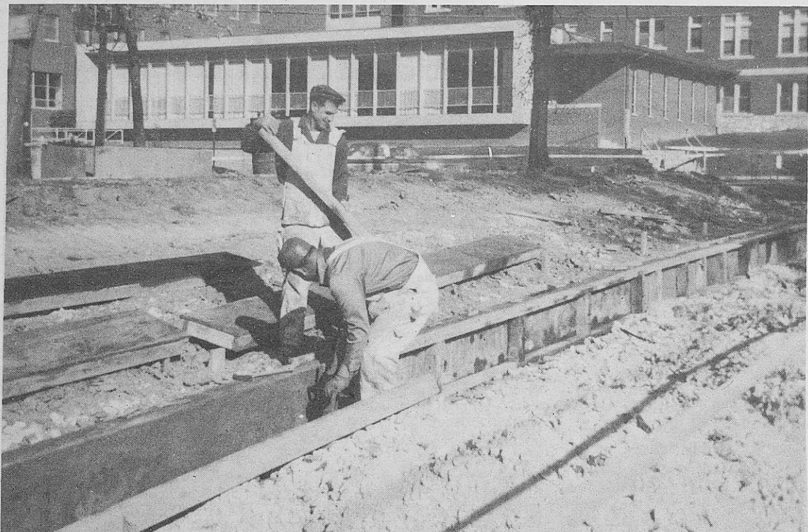
The corner of Big Bend Blvd. and Edgar Rd. is the current site for the activity of "Webster in Motion." Actually, they are widening the street for easy access to the new theatre. Part of the new look will be a pedestrian island, and part of the missing old look is a section of the wall surrounding the F.A.C.
