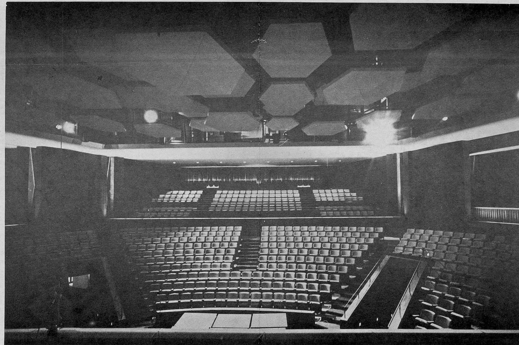
This view taken from the stage of the Loretto-Hilton Center for Performing Arts shows, on the lower right and left, actor's entrances to the thrust stage. These entrances, one sloping and one equipped with stairs, will allow actors to exit and enter from the front of the stage as well as from the wings. Visible at the top of the picture are the acoustical "clouds" which will distribute sound evenly throughout the theatre. And in the center, one of the auxiliary rooms, seating 250, is opened. This room and the bays to the upper right and left, will function as sound-proof classrooms when closed, but each room when opened will add from 125 to 525 additional seats to the auditorium proper.
