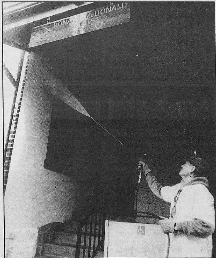
Mark Lesch, a computer science major, uses a power sprayer to clean the bricks of the Ronald McDonald House. Photo by Liz Streeter
