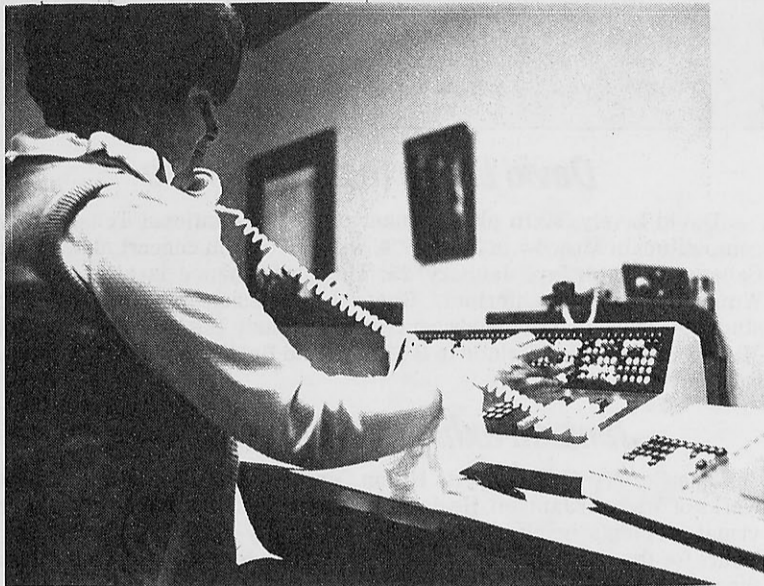
Charlotte Drapp, Webster's switchboard operator, at the helm of the new switchboard.
