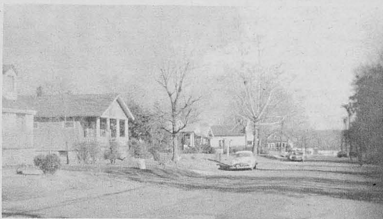
Although some houses in North Webster are obviously sub-standard, a number show signs of recent remodeling.
