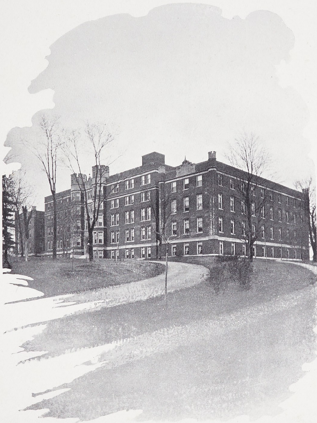
NORTH VIEW OF BUILDING
