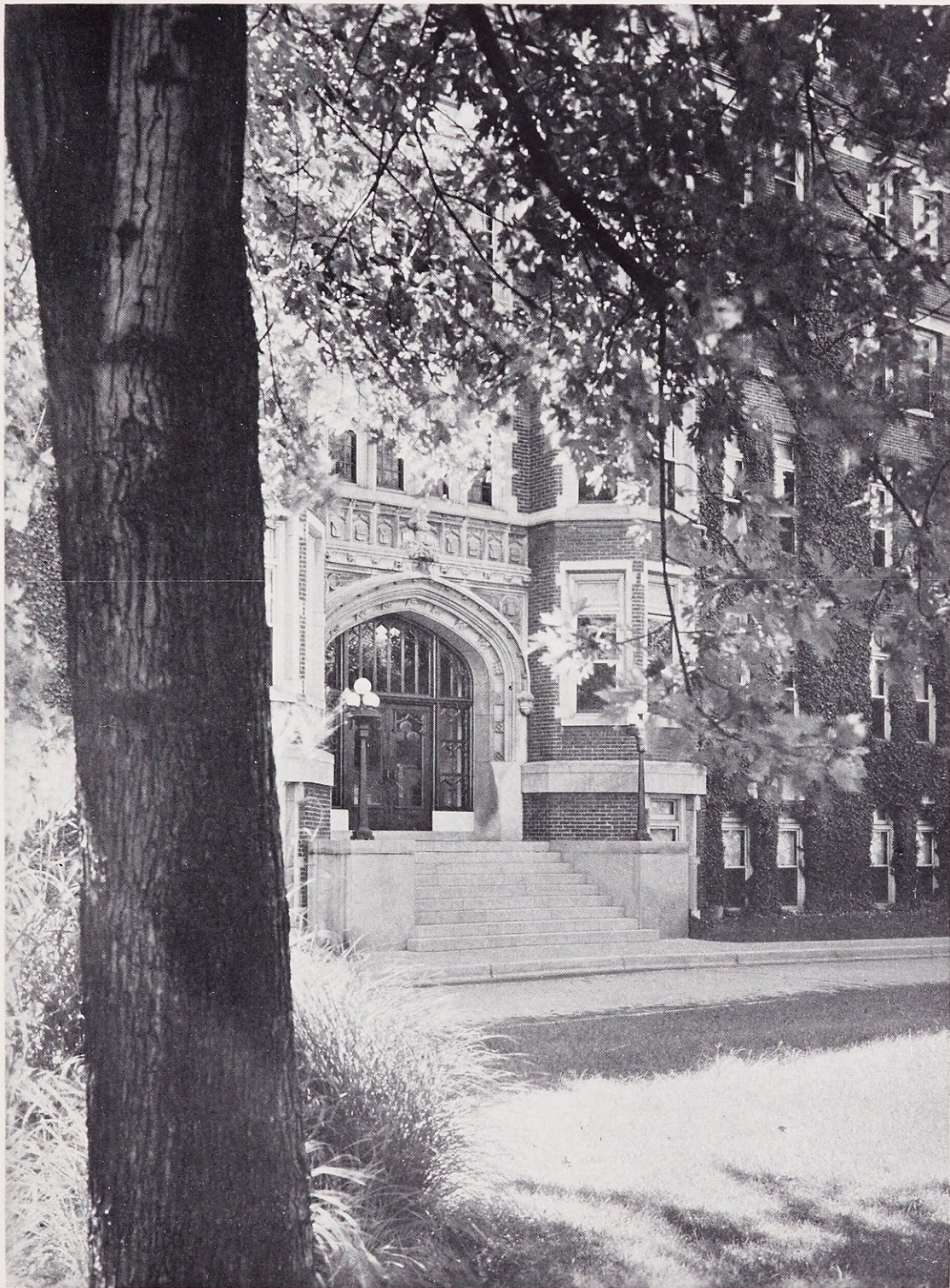
Front Entrance of the Administration Building.
