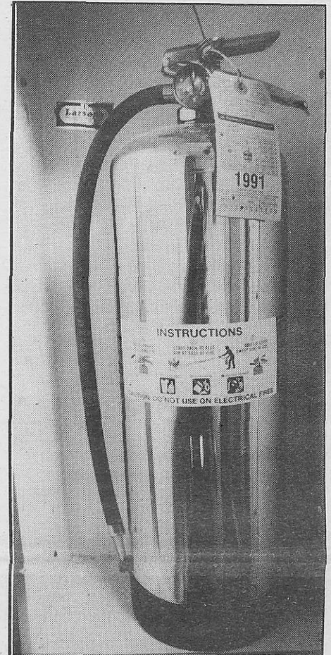
photo by Debra A. Robinson, The Journal This extinguisher is located behind the receptionist's desk in the Graduate Center.
