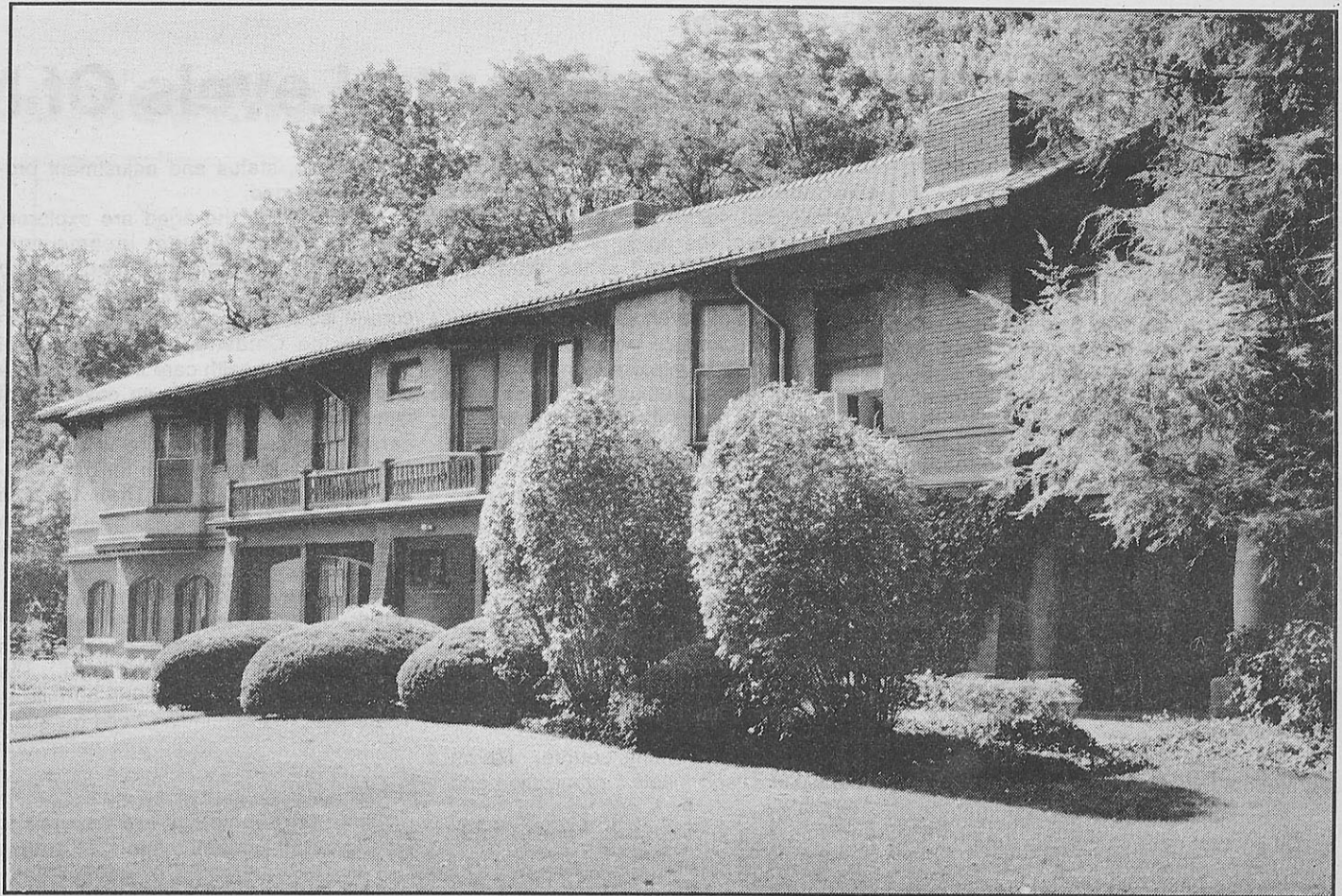
The Howe House, presently occupied, is mapped in phase 2 of Webster's development plan. photo by Mike Kornblum
