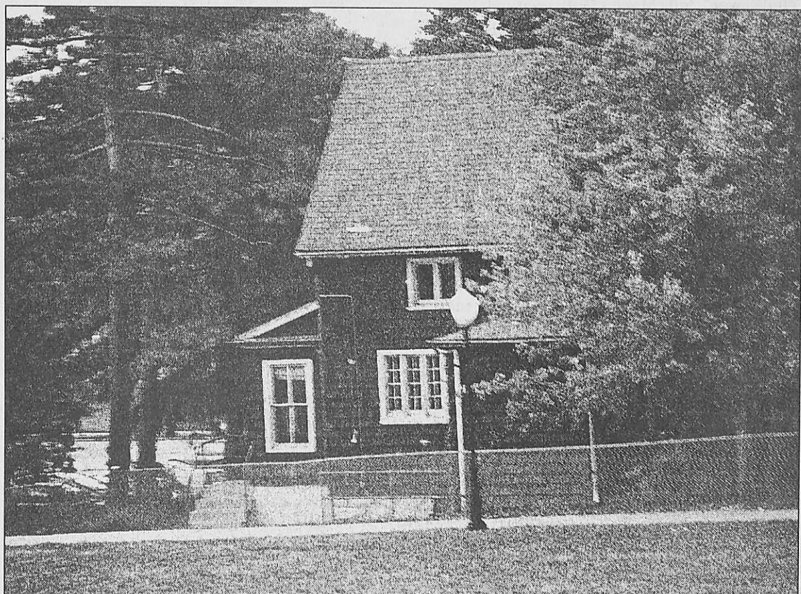
Jeff Starck/The Journal An orange construction gate encloses the Brown House, which will be demolished too make room for the library.
