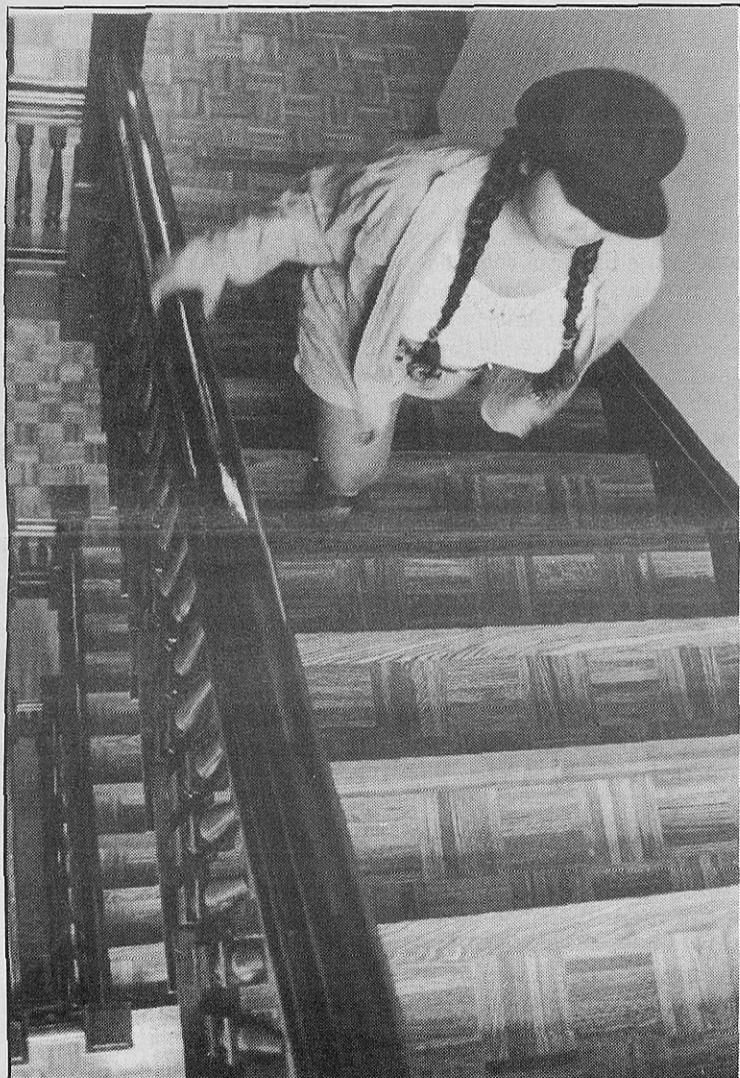
Webster student, Malia Arguello, uses the newly renovated stairs in Webster Hall. The stair treads were replaced with parquet flooring before the beginning of the '94 school year.
