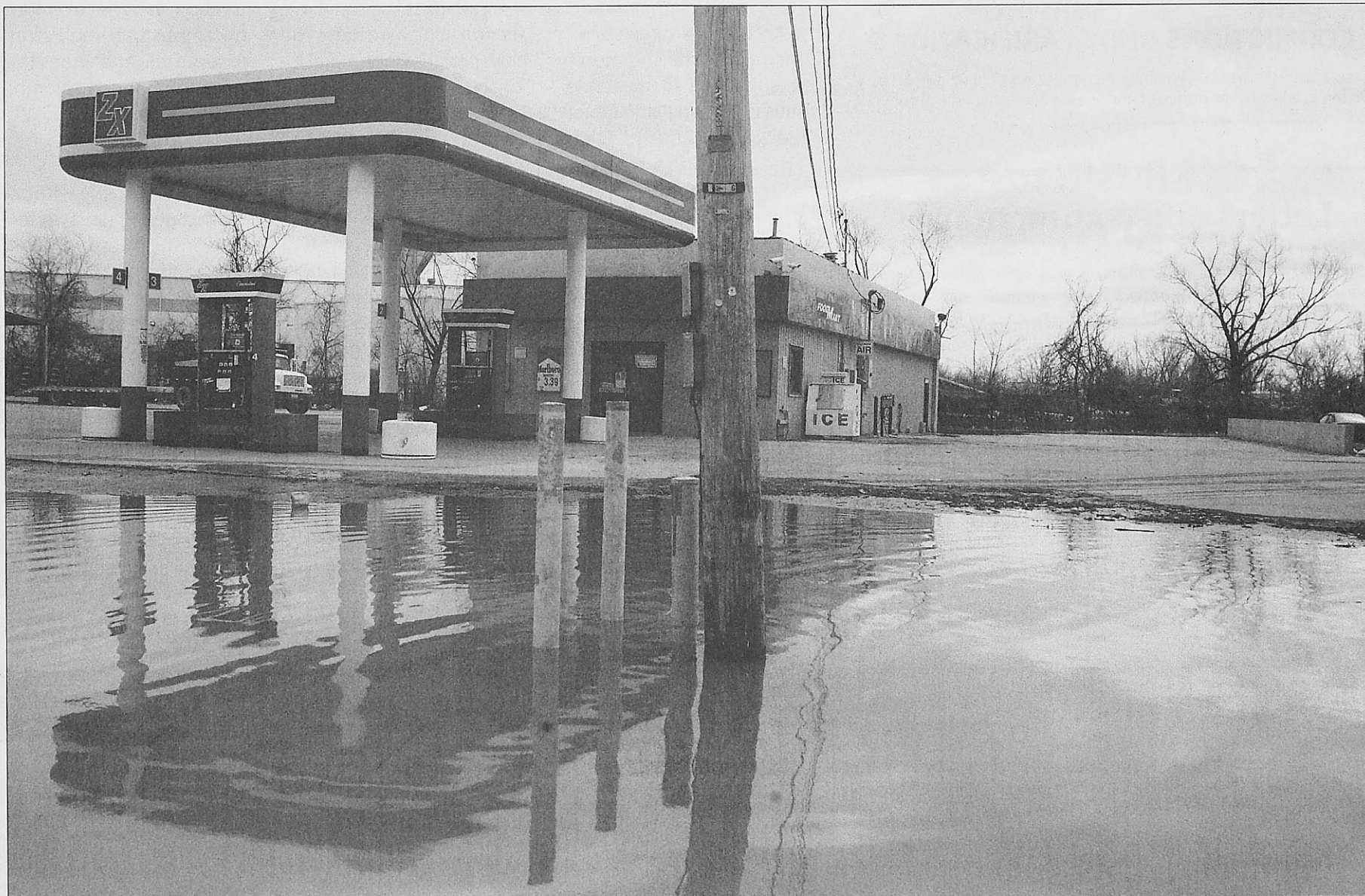
Floodwaters encroach on the pumps at the ZX gas station March 22 at the corner of Gravois and Rahning roads in Sunset Hills.
