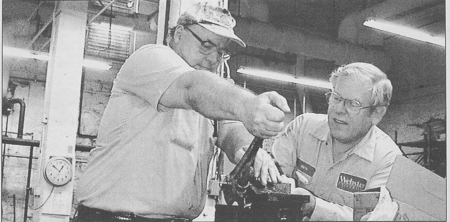
ABOVE: Ed Granich, left, and Ben Schaper make a repair in the physical plant on a piece of a broken toilet from the Sverdrup building on Oct. 13.
