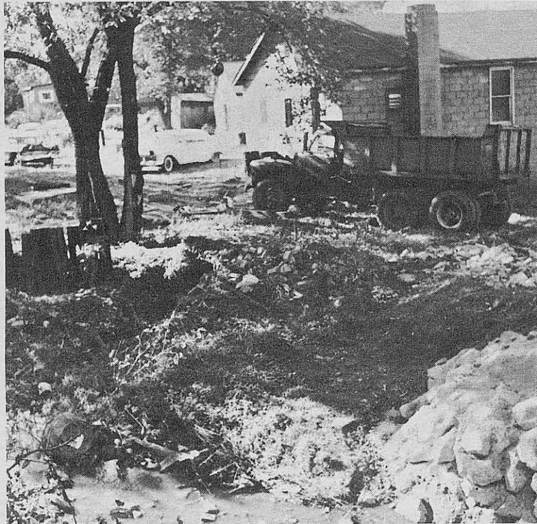
A Meacham Park home located next to an open sewer.
